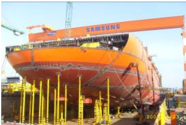
Aft section FPSO
